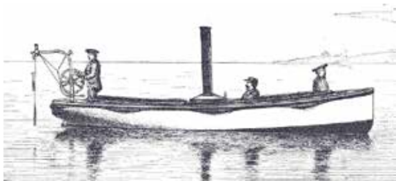
A sounding device from 1886
